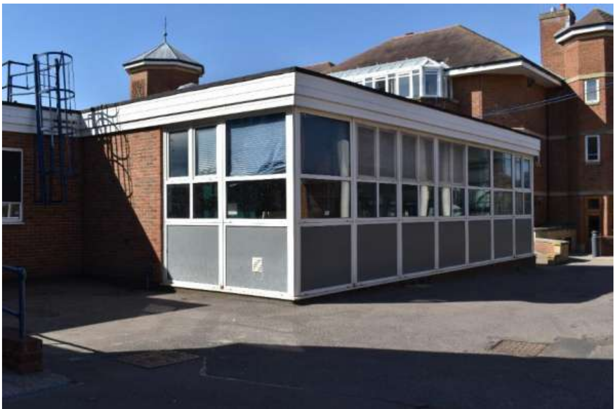
Plate 9: View of the old Kitchen to be demolished (facing NNW)
