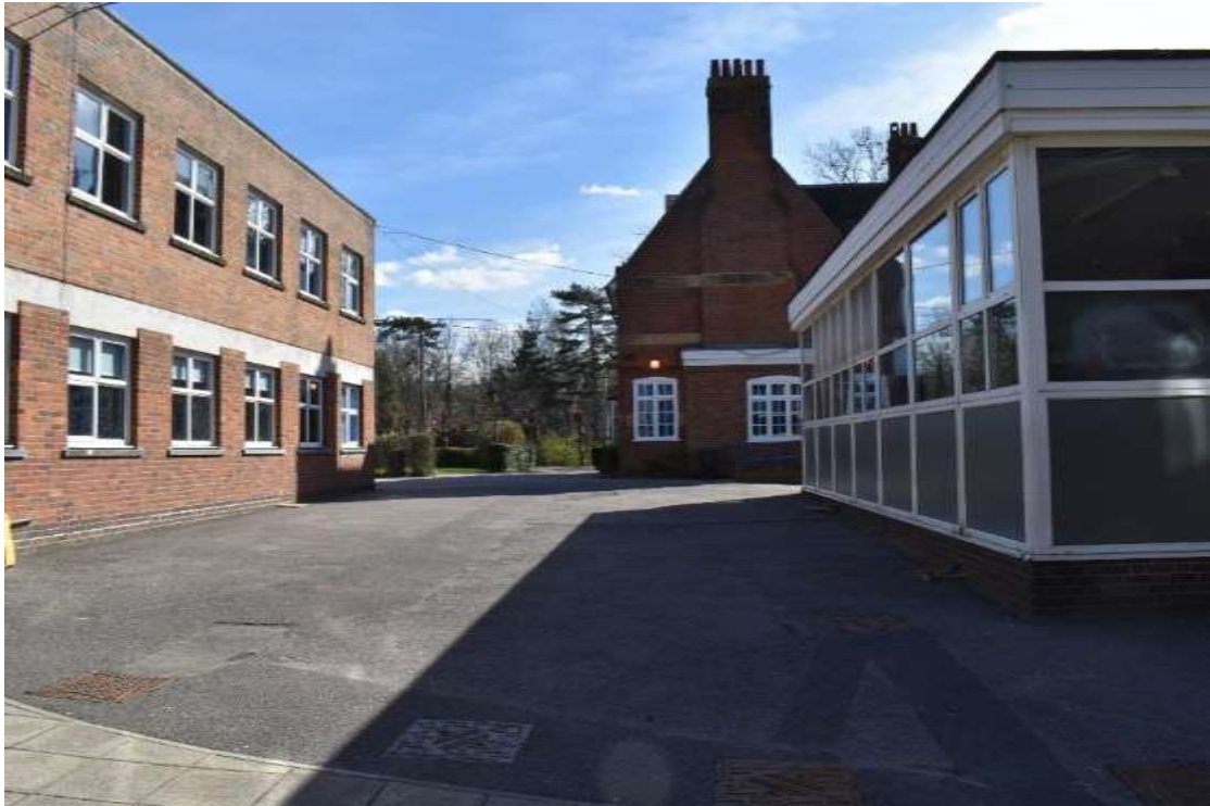
Plate 12: View of the RS block on the left and old kitchen on the right (facing SSE)
